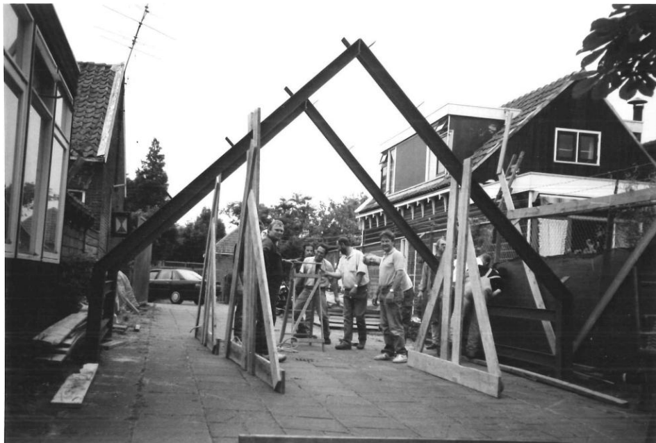
Figure 2 Local vernaculars: restoring green wooden house. Photograph from informant's collection.
